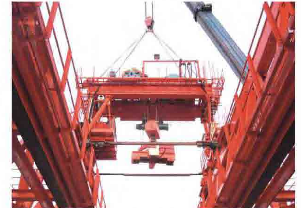
Installation of Winch Trolley
