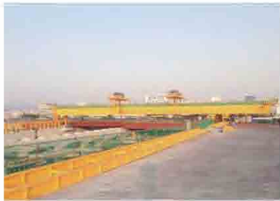
Beam Launcher for building Railway Station, Korea
