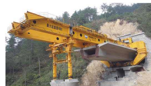
Girder-erection at Tunnel Portal
