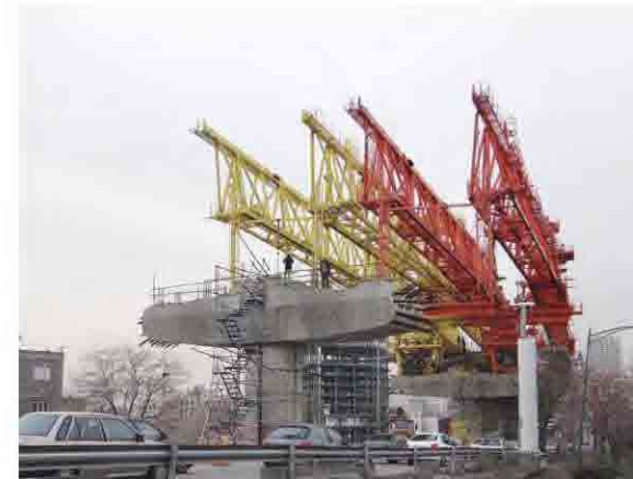
Girder Erection At Small Curve Section
